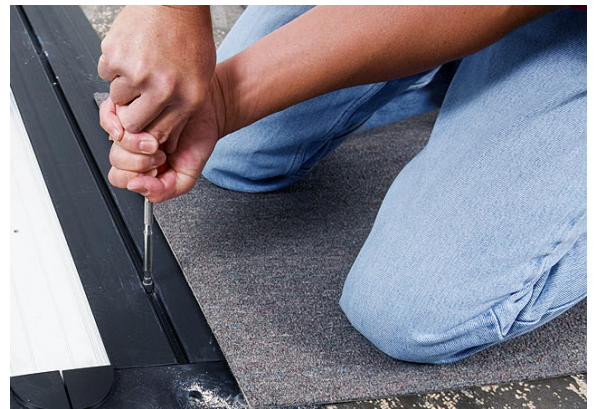
Screw side ramps to floor
